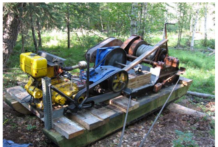
Winch used by project to pull wheel out of water at Rapids
